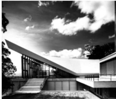
A friendly challenge to Nervi and Saarinen; structural elegance demonstrated with a parabolic vault. Jean Tschumi wanted to show his students the combination of concrete, steel, glass, brickwork, wood and linoleum in a realistic situation.
